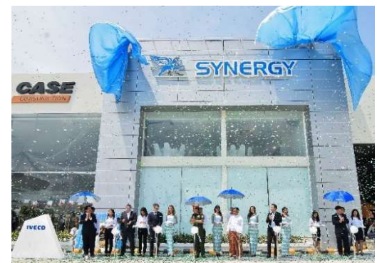
Headquarters cum commercial vehicles and construction equipment showroom – Myanmar
